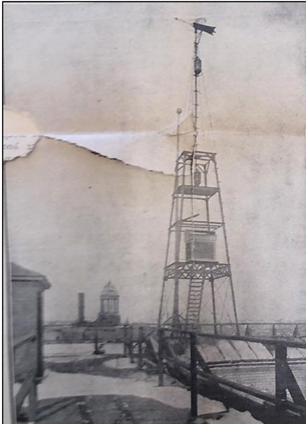
Figure 167. Iron tower on roof of Prudential Building showing wind vane and the instrument shelter (top of stairs) built into the tower. Image Source: Buffalo Illustrated Times, Clippings Book. Manuscript on file at Buffalo Museum of Science.
