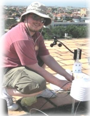
Matt Cutolo installing a meteorologic station on the roof of the Royal University of Phnom Penh.
